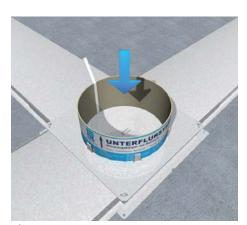
4 | Inserting the shuttering pipe
